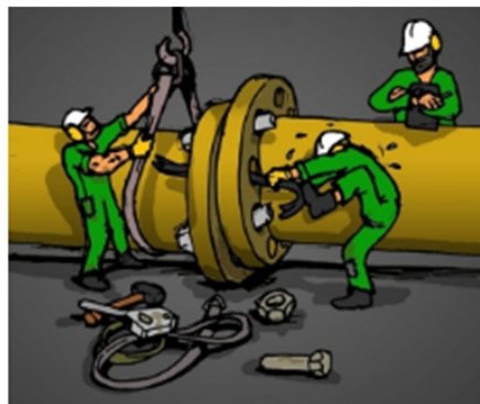
Traditional flange alignment method
