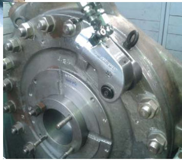
◀ PSD-3 Bolt tightening of Centrifugal pump casing
