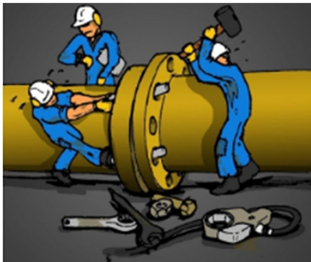
Traditional flange alignment method
